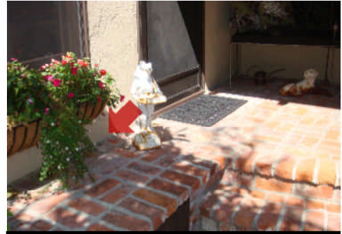
Surface appears level with interior floor.
