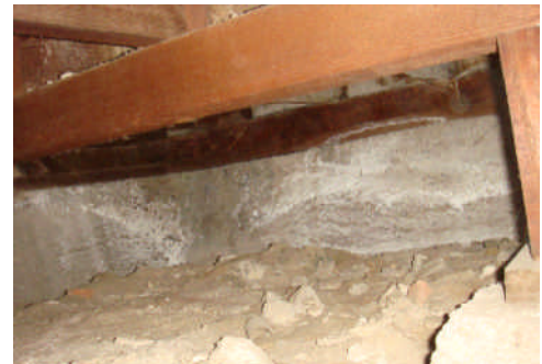
Foundation view at the rear left corner.
