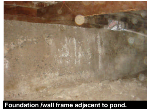
Foundation /wall frame adjacent to pond.
