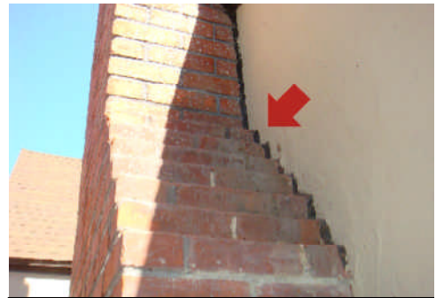
Mastic /tar appears to have been added.
