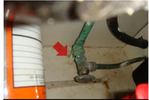
Water supply valve for dishwasher.
