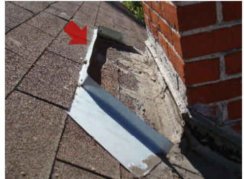
Seal chipped iron vent pipe.
