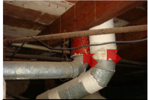
Water heater & abandoned furnace vent flue
