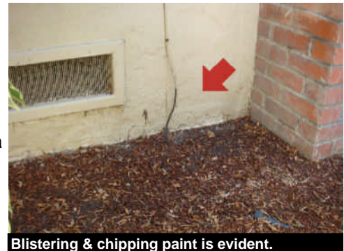
Blistering & chipping paint is evident.
