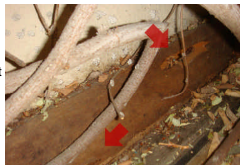
Insect damaged wood trim above window.
