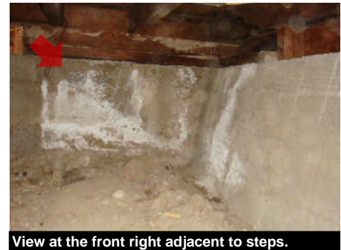
View at the front right adjacent to steps.
