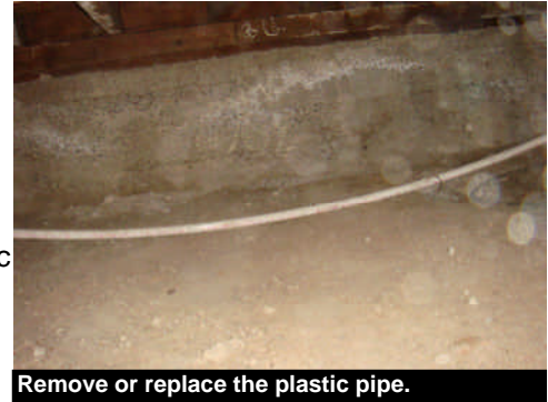
Remove or replace the plastic pipe.
