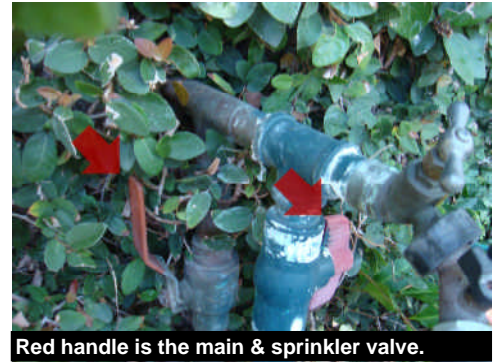
Red handle is the main & sprinkler valve.
