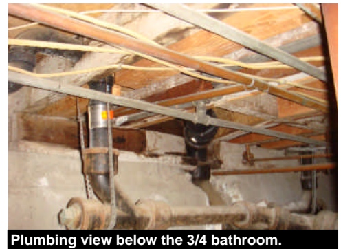
Plumbing view below the 3/4 bathroom.
