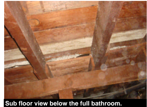
Sub floor view below the full bathroom.
