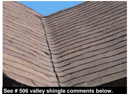
See # 506 valley shingle comments below.
