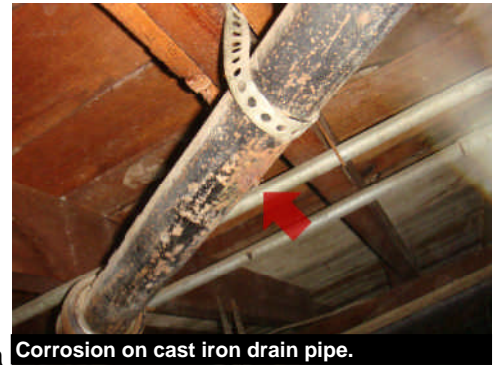
Corrosion on cast iron drain pipe.
