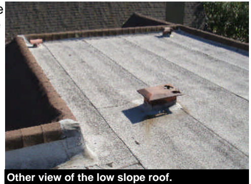
Other view of the low slope roof.
