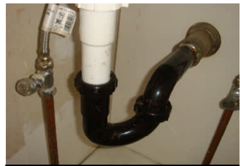
View below the 3/4 bath basin.
