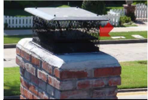
The damper operation should be evaluated.
