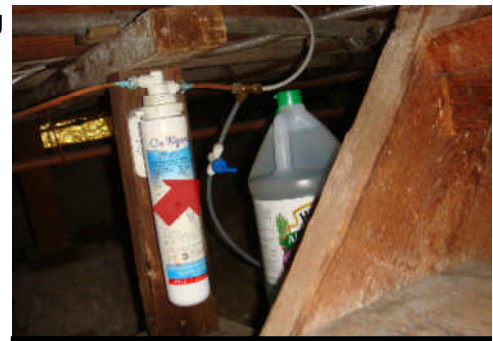
Filter in crawl space.
