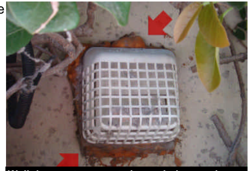
Wall does not appear to be sealed properly
