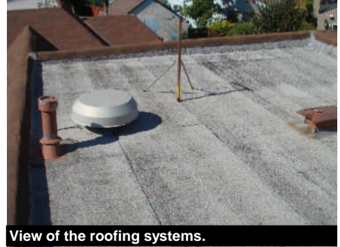
View of the roofing systems.
